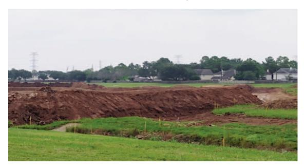
First Colony Levy Improvement District owns the property south of Lexington and west of Brightwater. Currently they have a 60-day project underway to increase the detention capacity of this area. The project entails removing dirt which will be used to bolster surrounding levy systems and in turn will allow more water to be held during heavy rain events. Water flow eventually drains into Oyster Creek. The land will be hydro-seeded after construction.
