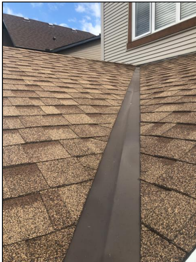
Roof upper garage
