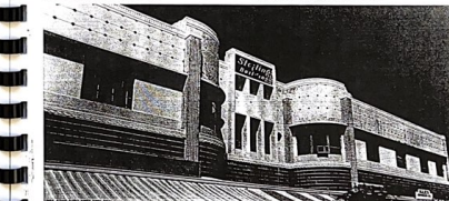
Horizontal window bands, glass block and sunshades are balanced against the vertical emphasis of the entry to the streamlined Sterling Building.
