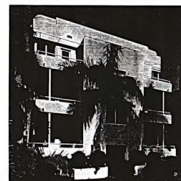
Horizontal recessed balconies counter the vertical center bay of this typical Art Deco block.
