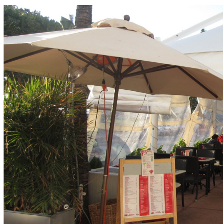
Electrical wiring or plumbing/ water lines
