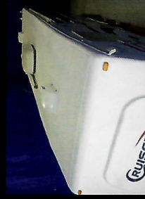
After picture with lifetime seamless caulk less roof.
