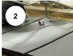
Lay the mats in the stalls a minimum of 2 inches apart. The gap is absolutely essential to allow for the expansion which occurs in the first few months. Don't worry about the gap filling with bedding...the Mayo Mat material is rigid enough that bedding does not work its way under the mat.
