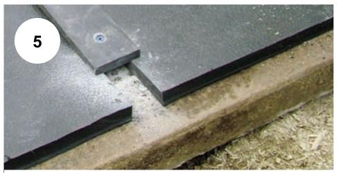
Fasten a "Mayo Plank" over the space between the mats. This is a 1 x 4 plastic board made from recycled plastic and rounded slightly on the edges. This keeps material from getting under the mat by preventing it from curling in very high intensity sunlight.
