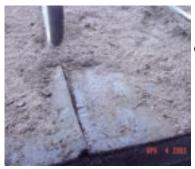
Also, a few mats may expand at the back corners as in this picture and start to touch each other. It is a good idea to slice out a wedge of each of these mats to restore the gap.
