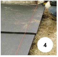
Finally, snap a chalk line down the entire row of mats 2 inches in from curb. See back panel for detailed cutting instructions.
