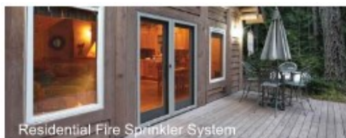
Residential Fire Sprinkler System
