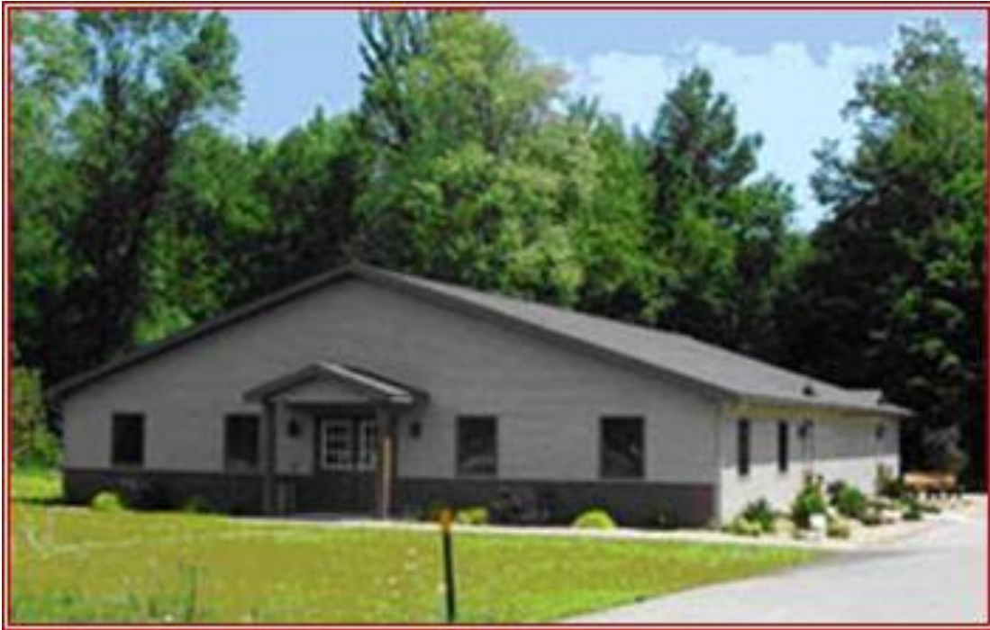
Figure 4.3 Secord Township Hall
