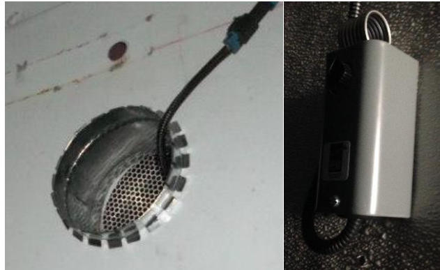
Figure 11: Remote thermostat installation
