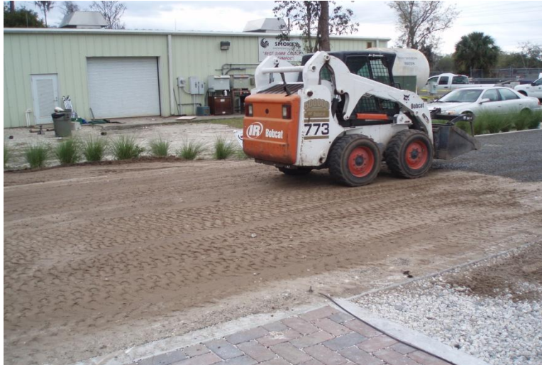
Figure 11: Spreading of A-3 sediments over the entire Rejuvenation section
