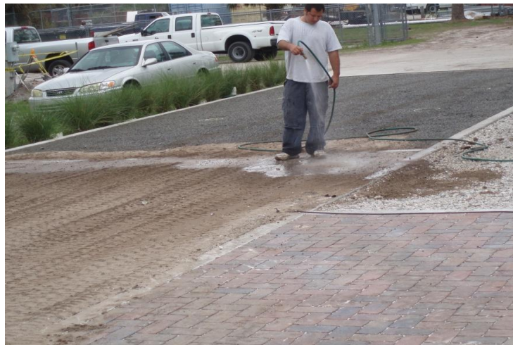
Figure 12: Washing sediments in with garden hose
