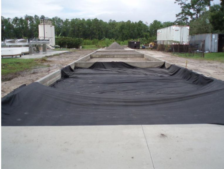
Figure 7: Filter fabric installed
