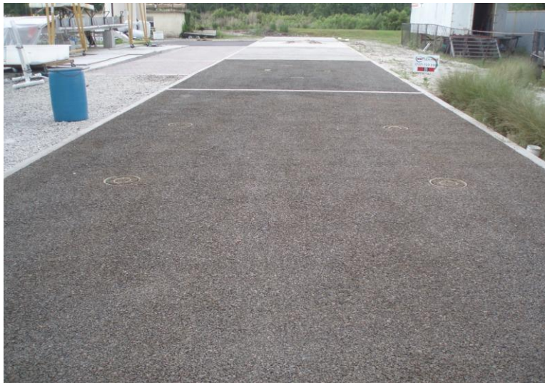
Figure 9: Final layout of FlexiPave sections
