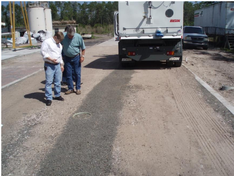
Figure 16: ERIK test after sediment loading
