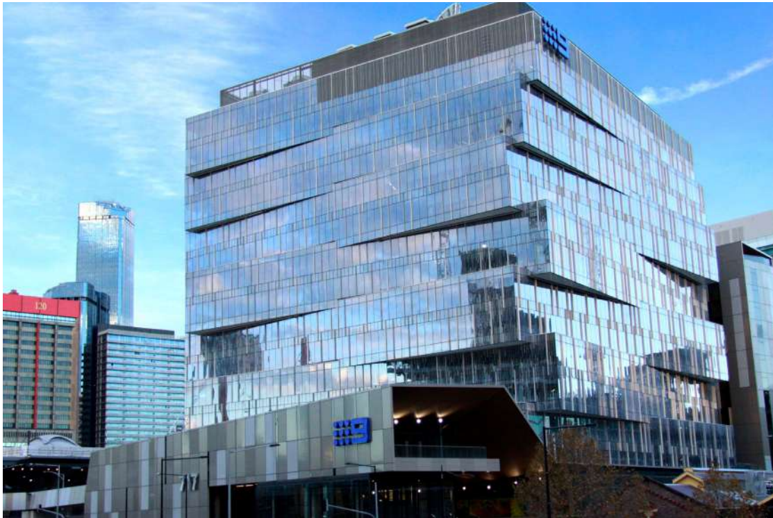
717 BOURKE STREET, MELBOURNE Product: DGU Double Silver Low-E Coating on Clear Glass; Laminated Glass; Clear Glass with Colourback coverage
