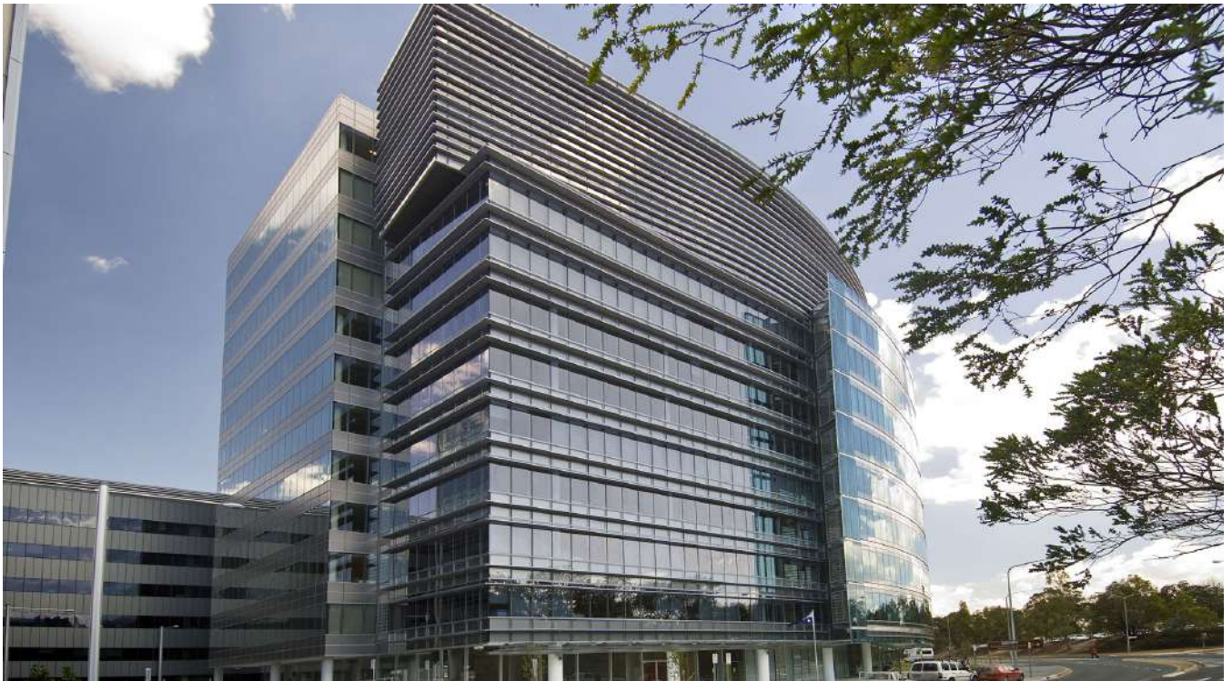
18 MARCUS CLARKE, CANBERRA Product: DGU Double Low-E Neutral Coating on Clear Glass; Clear Laminated Glass
