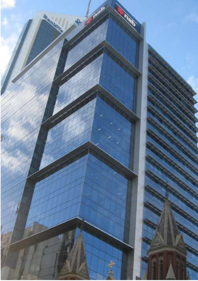
CENTURY CITY, PERTH Product: DGU Double Low-E Coating On Dark Blue Tinted Glass
