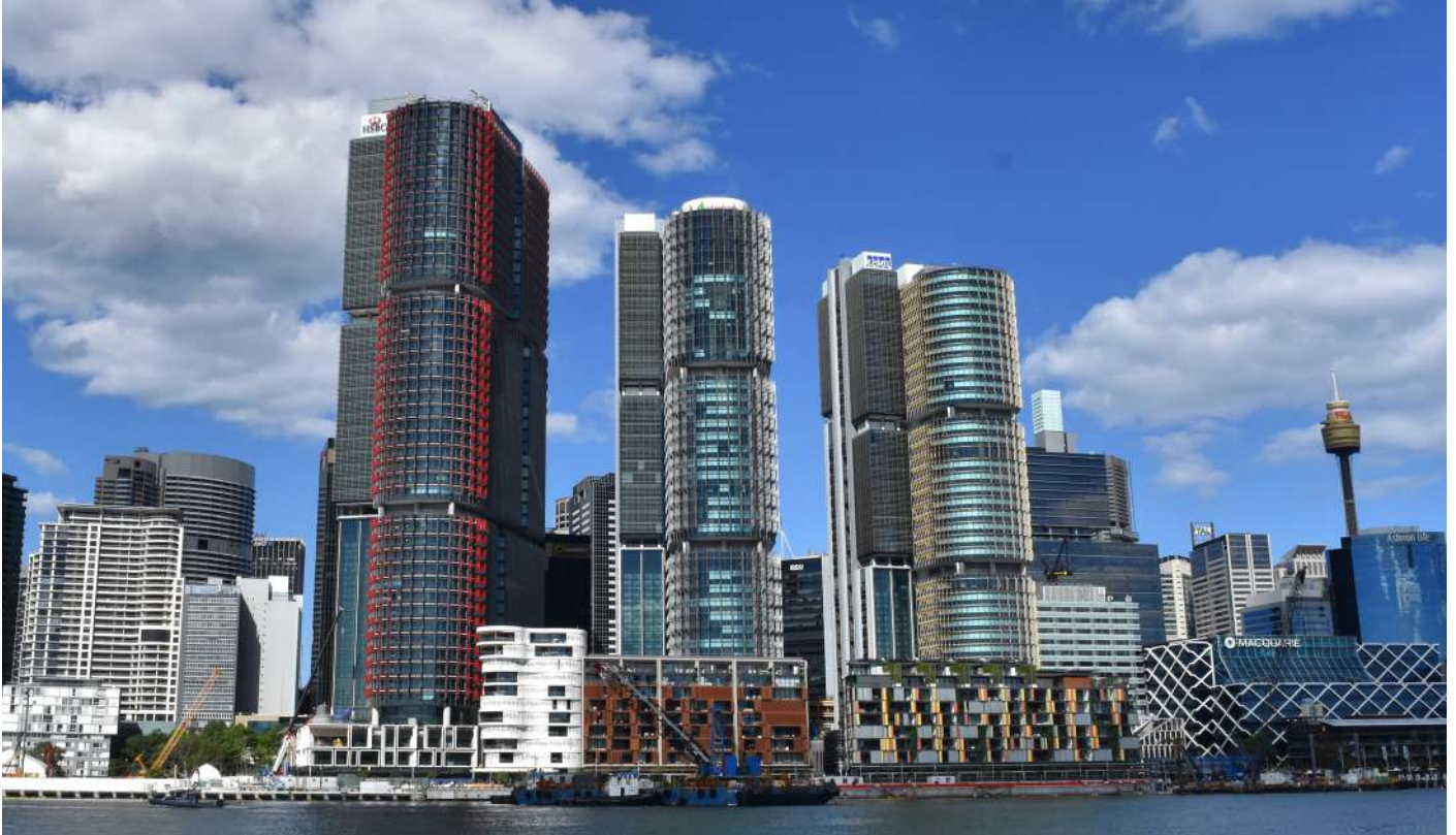
INTERNATIONAL TOWERS SYDNEY, BARANGAROO Product: DGU Triple Low-E Neutral Coating On Clear Glass
