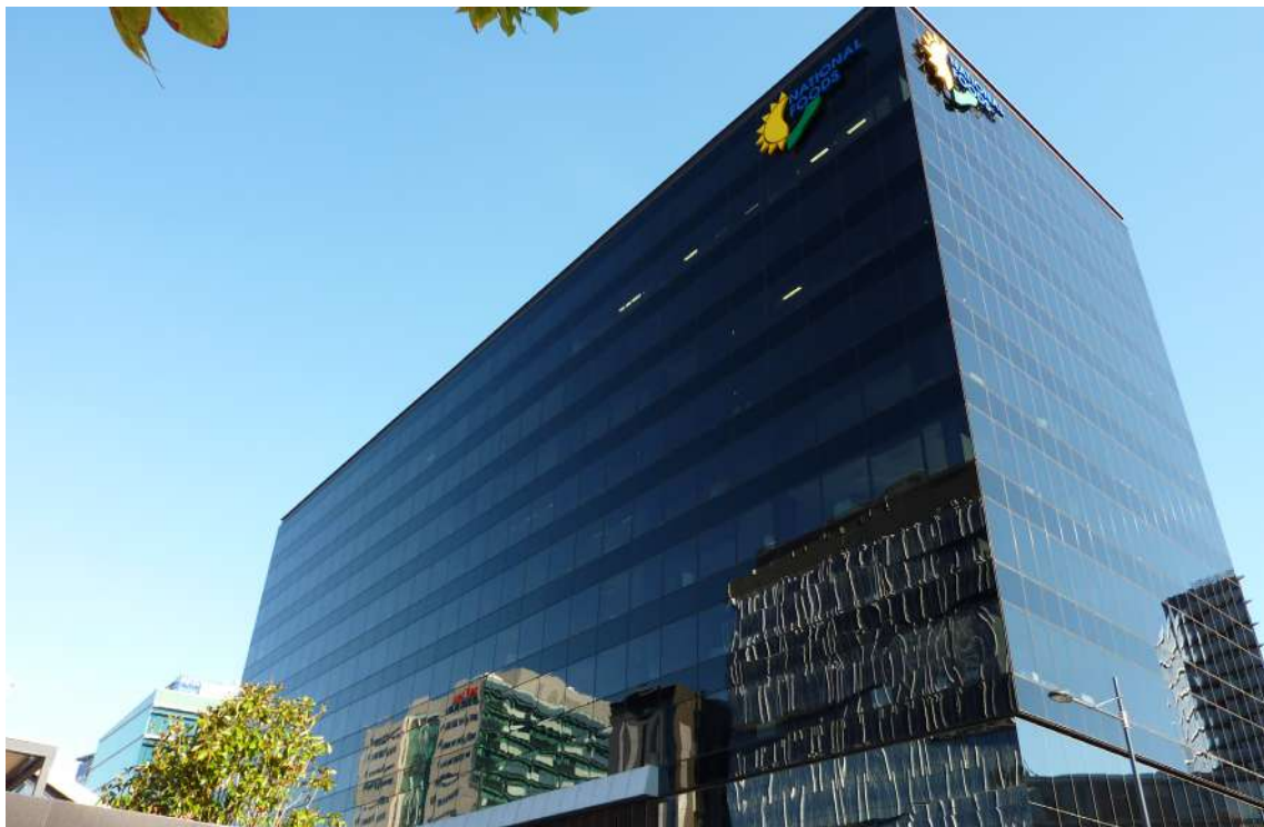
737 BOURKE STREET, MELBOURNE Product: Grey glass with Ceramic Frit; DGU with Low-E Coating and Solar Reflective Coating on Clear Glass
