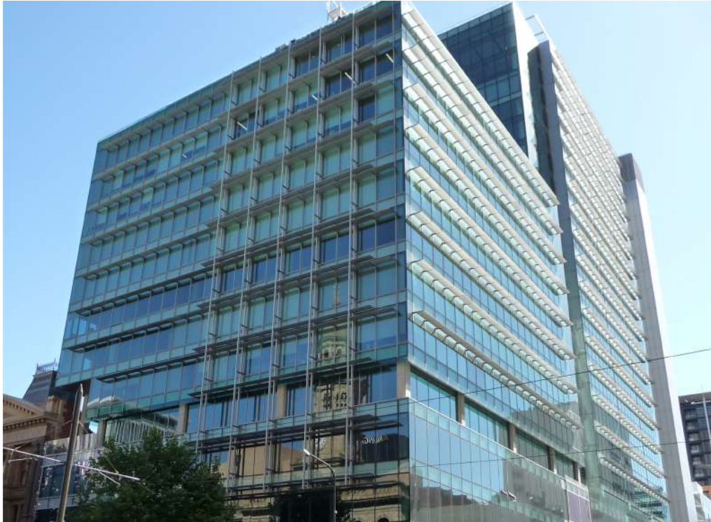
CITY CENTRAL TOWER, ADELAIDE Product: DGU Double Low-E Coating With Green Tinted Glass
