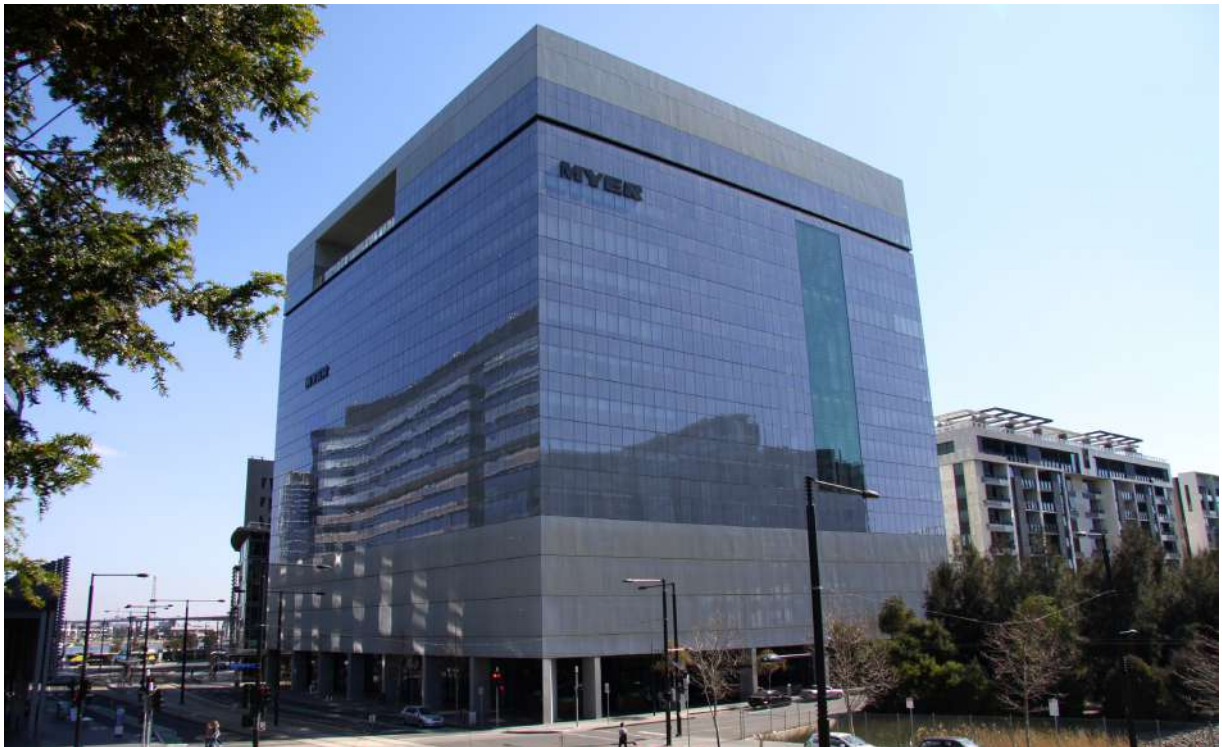
800 COLLINS STREET, MELBOURNE Product: DGU Double Low-E Neutral Coating With Clear Glass
