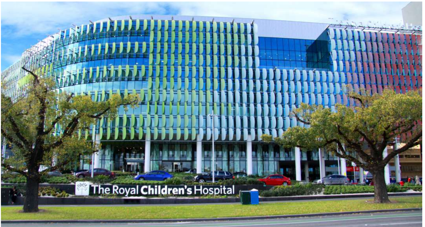
ROYAL CHILDREN'S HOSPITAL, MELBOURNE Product: DGU Double Low-E Coating On Green Tinted Glass; Laminated Glass Pink, White, Green Colourback With Performance Glass
