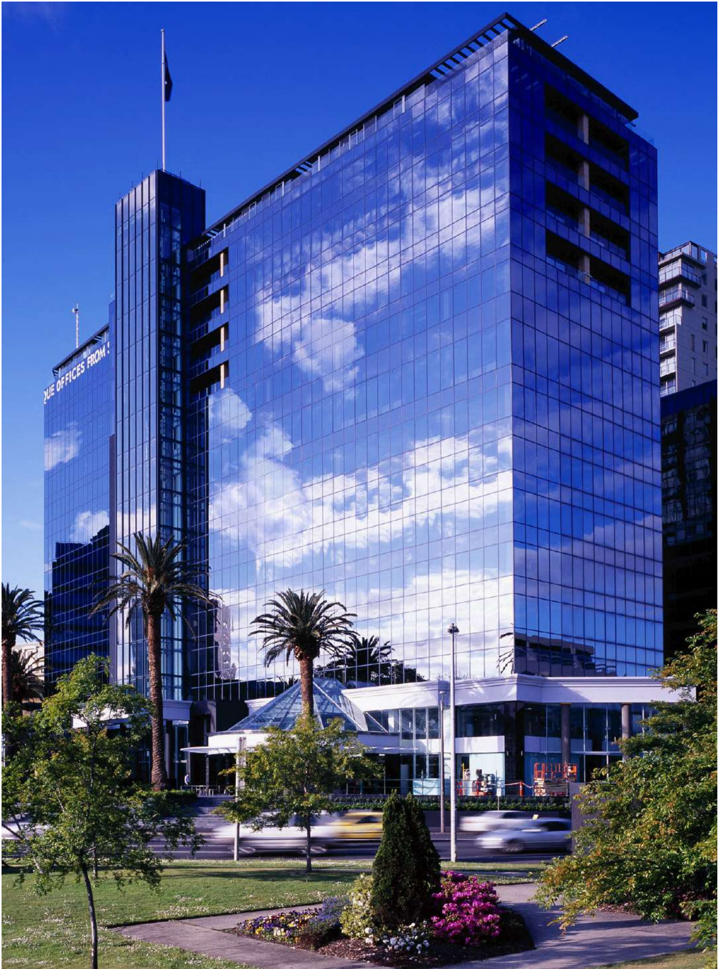
ST KILDA ROAD TOWER, MELBOURNE VIC TOTAL FAÇADE AREA: 4000M2 | PRODUCTS DGU GLASS WITH SOLARPRO SOLAR REFLECTIVE COATING
