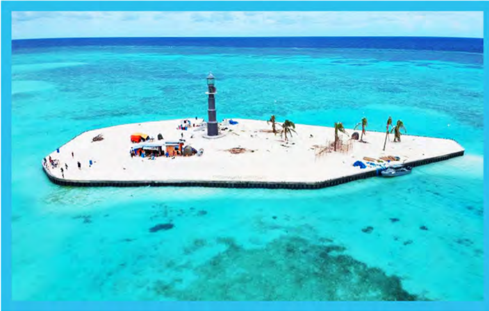
Figure 2. A new structure to replace the 40-year old lighthouse in South Atoll was completed in June.
