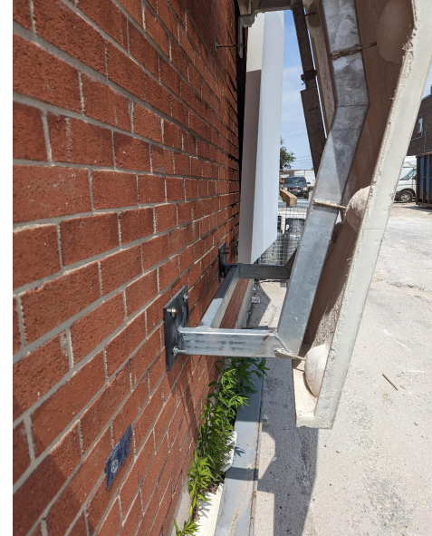
Image: testing Elise Tower podium spandrel panels by Petra Design
