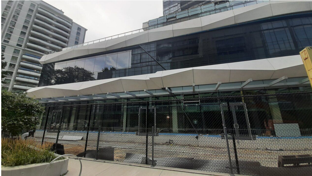
Commercial Tower Cladding LARGE SCALE GFRC EXTERIOR CLADDING Fabricated by: Petra Design, Toronto
