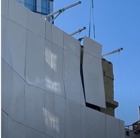
Commercial Tower Cladding LARGE SCALE GFRC EXTERIOR CLADDING Fabricated by: Petra Design, Toronto
