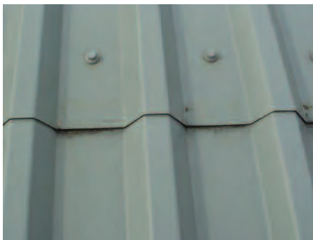
Colorcoat HPS200 Ultra® with Galvalloy® roof after 7 years.
