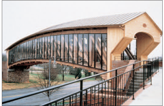
Old Salem Covered Bridge; Winston-Salem, North Carolina (courtesy of Blue Ridge Timberwrights)
