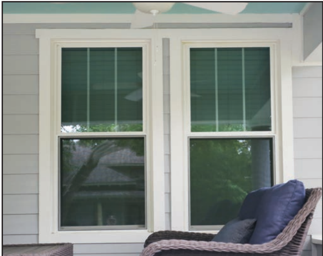
Three-over-one windows (energy efficient)
