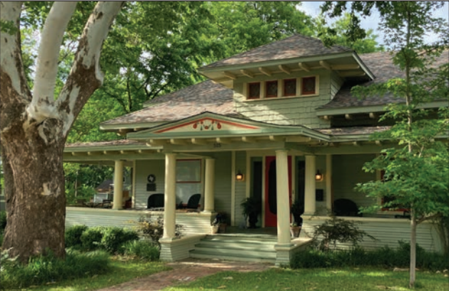
515 W. Hunt Street (Burton House)
