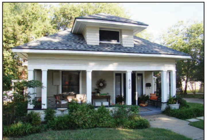
The centrally located dormer is a hallmark of the American Foursquare Style. While the dormer implies a living space, it was more often framing a slatted wooden vent intended to ventilate an uninhabited attic. The American Foursquare used porch space as a defining element that had the practical advantage of providing a comfortable sitting area in warmer weather.
