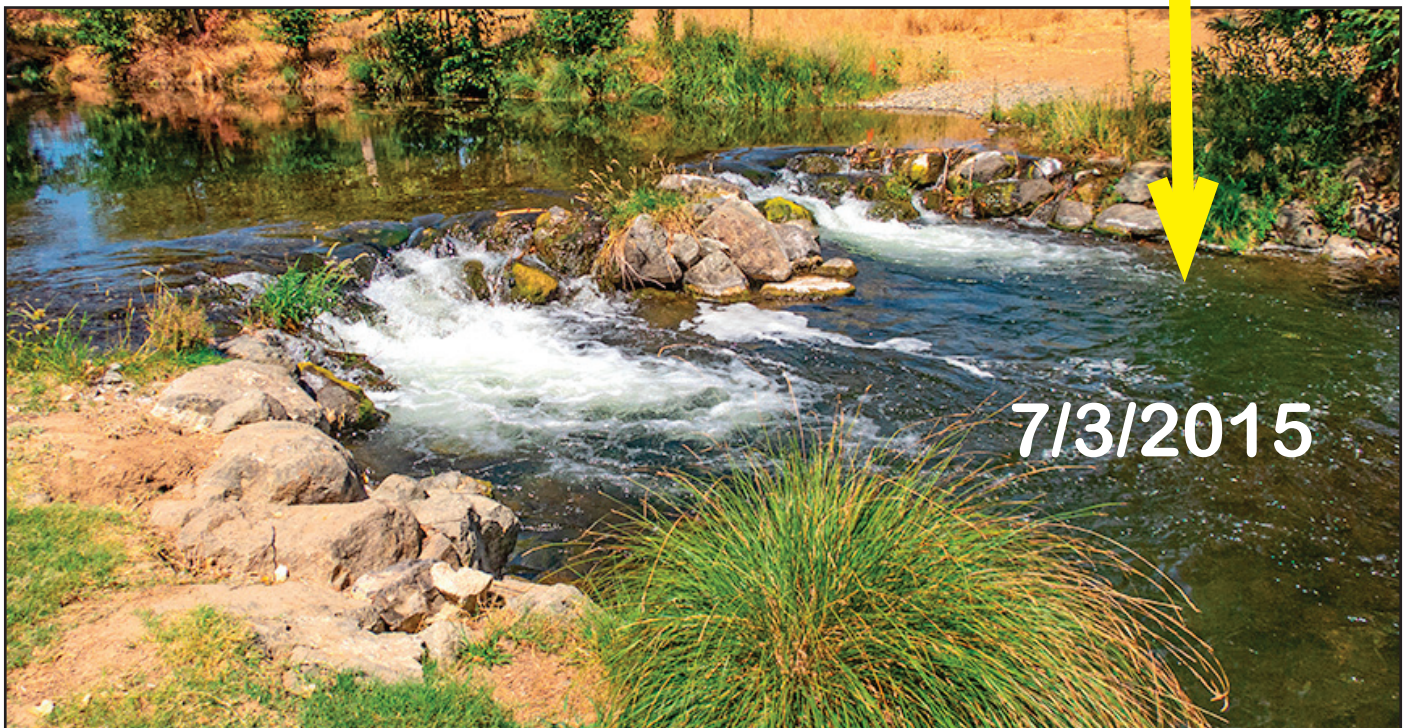
Image taken 7/3/2015: The Pickrel Weir was constructed in 2009. The natural scour just below the weir created a situation similar to mechanical scarification that has proven beneficial for salmon spawning. Information suggests that several salmon spawned in the small section in 2012 amid a sediment-laden waterway. They were undetected. The following spring, thousands of juvenile salmon were found 75 feet downstream (and much further) from the weir on May 1, 2013. I have also documented that the weir had a very positive effect on benthic macroinvertebrates. Ken W. Davis image
