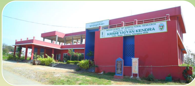
EGVF-KRISHI VIGYAN KENDRA ADMINISTRATIVE BUILDING
