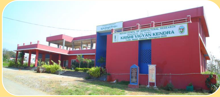
EGVF-KRISHI VIGYAN KENDRA ADMINISTRATIVE BUILDING
