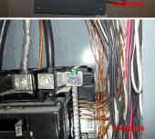
Repair or Replace Service Entrance Cable: Aluminum service entrance - Needs to be properly secured to the home.
