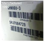
Type: Forced air Capacity: 60,000 BTU Approx. Age: 1994 / 29 years old Area Served: Whole house Fuel Type: Natural gas Suspected Asbestos: No Repair or Replace Heating System
