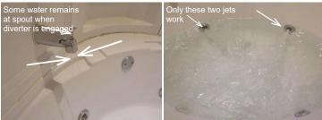
Limited Inspection Tub Plumbing: Tub drained okay - No access to tub motor. No access panel to tub faucet plumbing. Plumbing was viewed from the basement only with no issues noted from that view.
