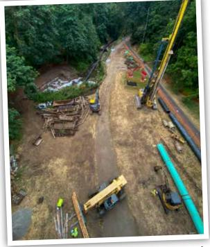
The Bureau of Development Services is replacing the wooden trash rack over Balch Creek in Lower Macleay Park, where the stream is diverted into a culvert that empties into the Willamette River. Photo by Matt Erceg
