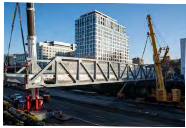
The Flanders Crossing Bike and Pedestrian Bridge was installed Jan. 23 using two giant cranes. The bridge will complete a neighborhood greenway linking Northwest Flanders Street between 24th Avenue and the Willamette River. Traffic signals will be placed at 14th and 16th avenues and four-way stop signs at 15th Avenue. Opening is promised “by this summer.”
