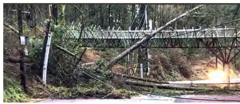
A landslide on West Burnside Street on Jan. 12 knocked over about six large trees, destroying power poles and covering the street with enough debris to fill 42 dump trucks. The street was closed for a week. Engineers are assessing possible damage to the Barbara Walker Crossing caused by a falling tree.
