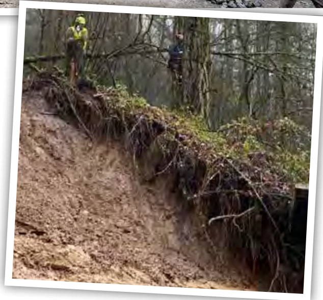
A landslide on West Burnside Street on Jan. 12 knocked over about six large trees, destroying power poles and covering the street with enough debris to fill 42 dump trucks. The street was closed for a week. Engineers are assessing possible damage to the Barbara Walker Crossing caused by a falling tree.
