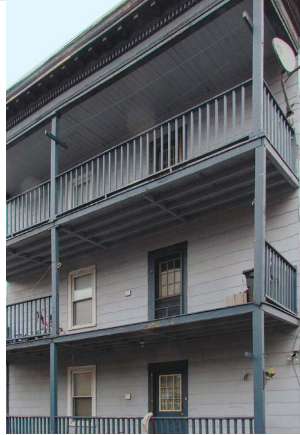
Toenailed railing-to-post connection fails. Over time, the wood decayed and the nails rusted. The weakened railing fell to the ground when someone leaned on it.
