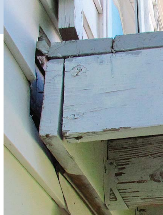
Detaching ledger. In this case, the homeowner noticed the failure of the nailed connection before the deck gave way. In other cases, decks have given way suddenly, often when they've been loaded with people.
