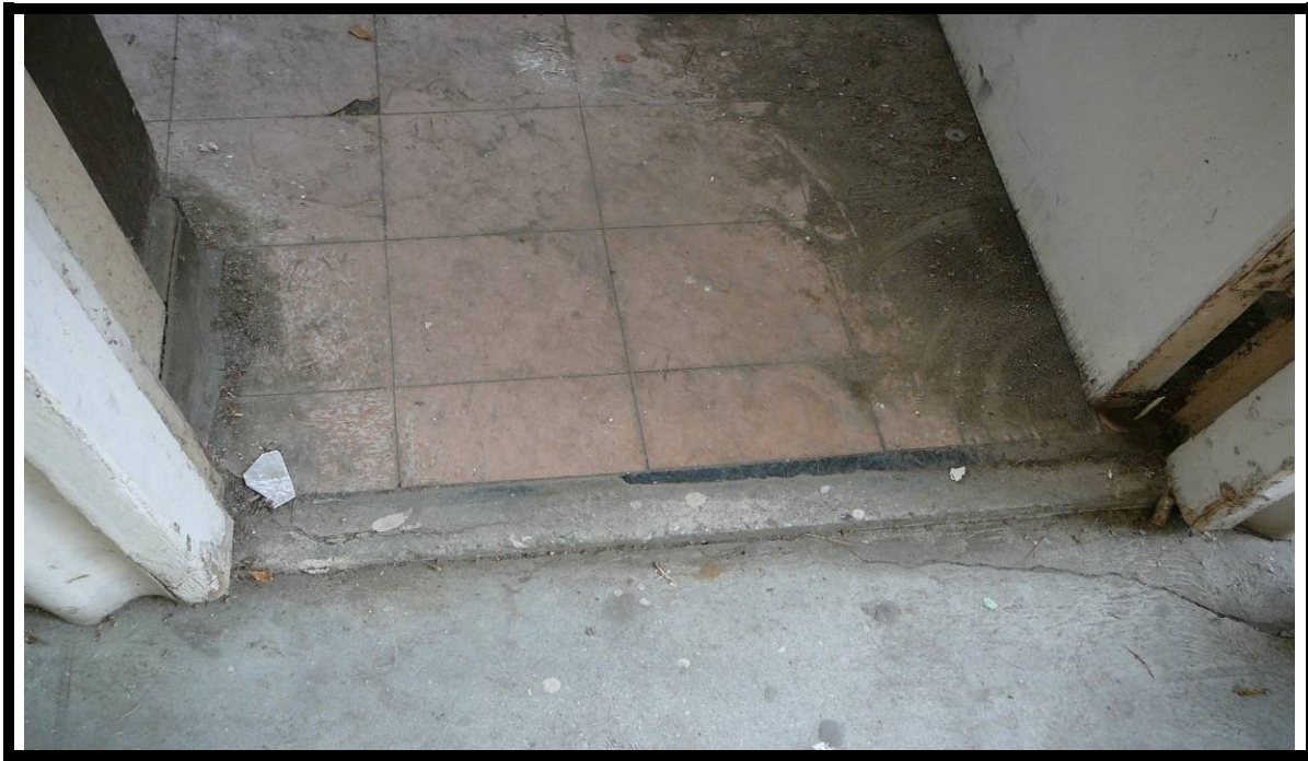
Photograph 1: View of the 9-inch by 9-inch asbestos containing vinyl floor tiles located in the “office” structure at the Community Building.
