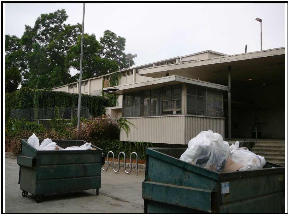
Photograph 4: View of the Community Building located at the El Sereno Recreation Center.
