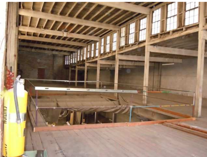
Construction area in the CAAH
