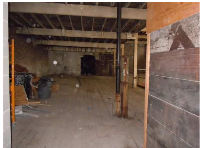
Construction area in the CAAH
