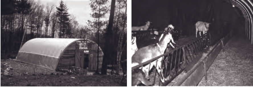
Figure 17.5 Low-cost hoop buildings with feeding alley adjacent to fabric wall (Ray Rodriguez, Rindge, NH). Courtesy: John C. Porter, Professor and Dairy Specialist, University of New Hampshire Cooperative Extension, www.umaine.edu/animalsci/Sheepgoats/Dairy%20Goat%20Housing.ppt . For color detail, see Appendix A.
