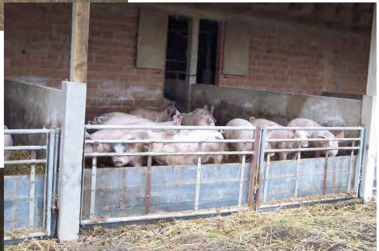
The grower/finisher pen is open sided for plenty of natural daylight and ventilation
