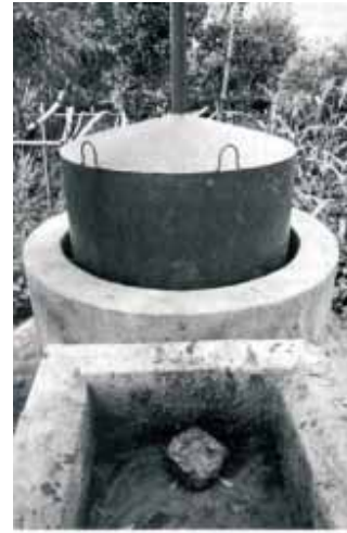
Plate 1 Biogas plant, example from India.
