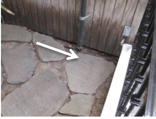
(north exterior of the guest house)
