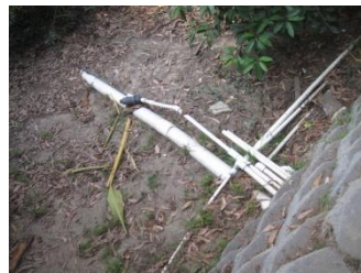
(south exterior of the guest house)
