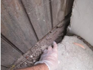
(north exterior of the guest house)
