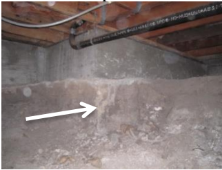
(one area under the back left of the building)
