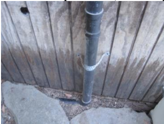
(north exterior of the guest house)
