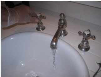
(jack-and-jill bathroom – downstairs)
