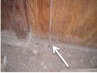
(main house crawlspace near the crawl entrance)
