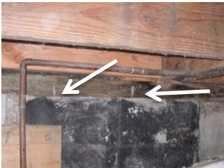
(e.g., north side of the guest house building)
