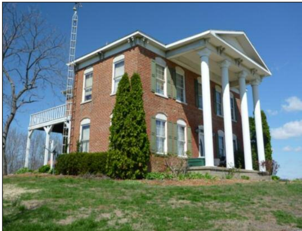
-Photo provided by the Indiana Division of Historic Preservation and Archaeology The Starlin Sims House, located on Hwy. 231 in Perry Township was built around 1850.
