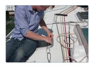
$12\,$  Feed the intended line or halyard into the textile sleeve using the splicing fid.
