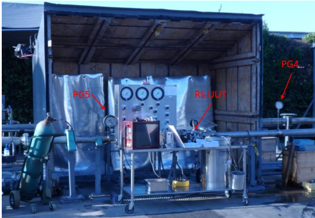
FIGURE 60 CLOSING RESPONSE WITH FLOW: WATER FLOW TEST STAND
