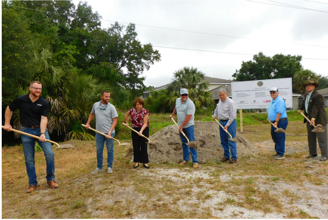
The City held a ground-breaking for 12th Ave. on April 22: from left, Brian Crowl of DRMP providing Construction Engineering & Inspection (CEI) Services for the project; Chad Baker, Project Manager for Andrew Sitework; Assistant City Administrator Beth Carsten; Public Works Director Steve Underwood; Deputy Major Keith Keene, Mayor Bob Heine, Jr., and City Administrator Terry Stewart.
