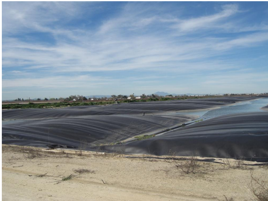
Fig. 10: Anaerobic lagoon digester at Castelanelli Brothers Dairy (Source: Authors own)
