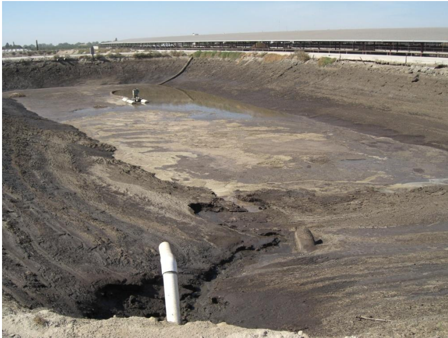
Fig. 9: Liquid digestate storage in a lagoon prior to land application at Fiscalini Farm (Source: Authors own)
