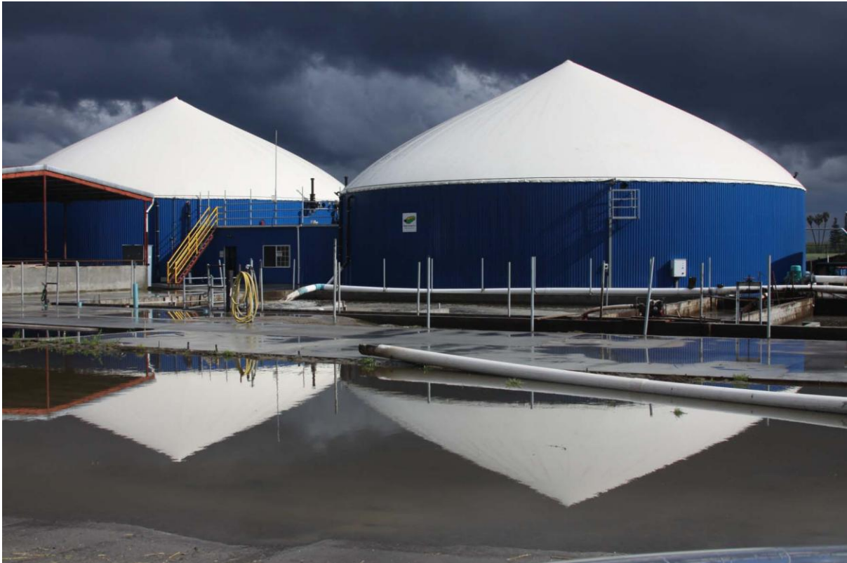
Fig. 7: The two mesophilic anaerobic digestion tanks at Fiscalini Farm (Source: Nettie Drake)
