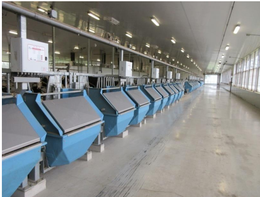
Recent installed feed intake facilities at the University of Guelph
