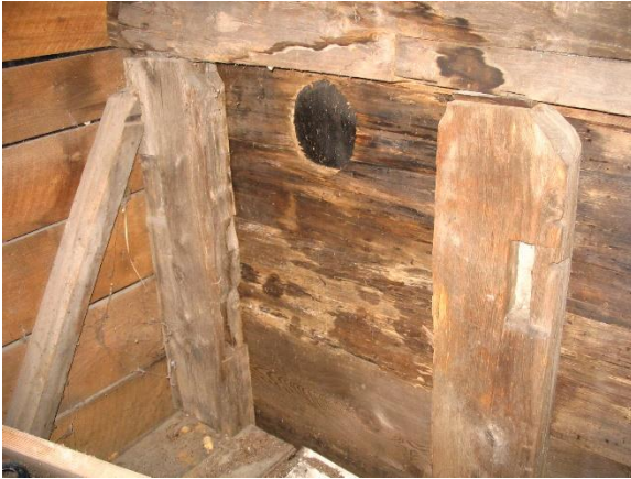
The structure of Rod Jessup's garage.
