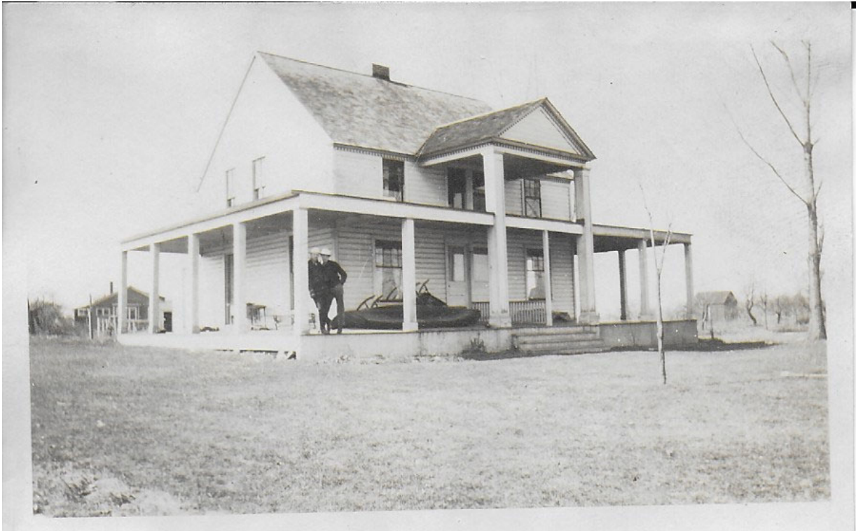
Thomas Roger and Alfred E. D. Allen on the porch of the duplex house built for the two families.
