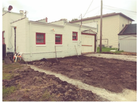
2. Foundations are poured
