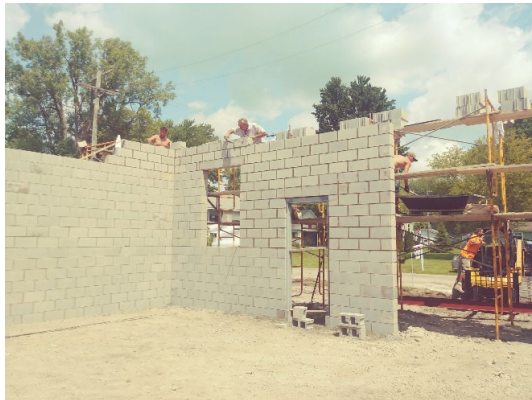
3. Masonry walls are erected
