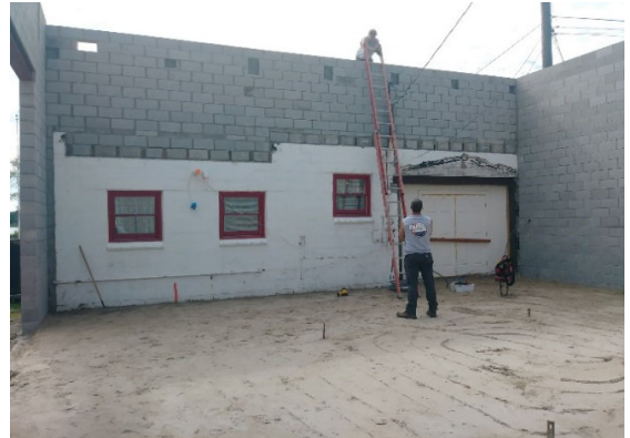
4. Sand base for floor brought in
