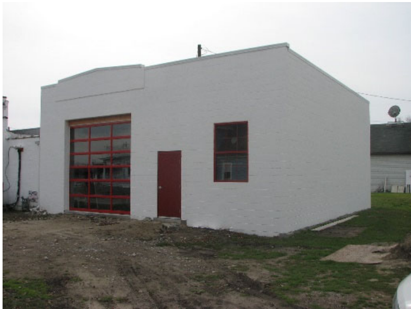
9. The exterior is painted, and windows and doors are installed
