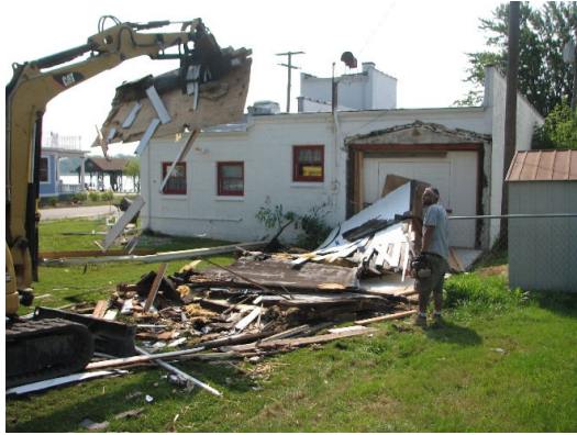
1. The old storage structure is removed
