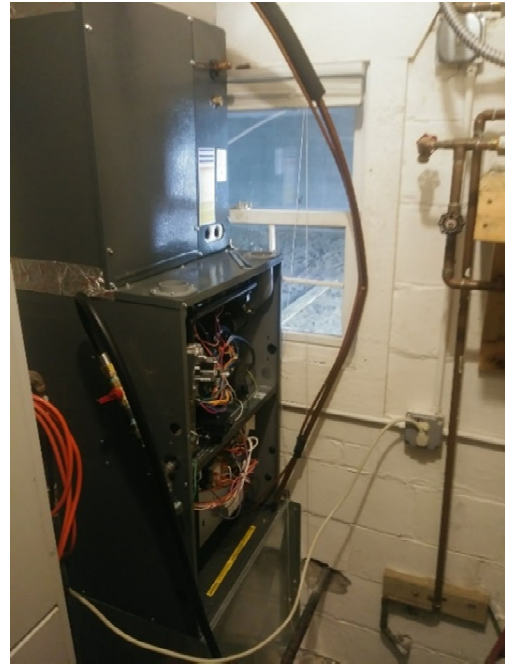
8. Heating and air conditioning 85% complete
