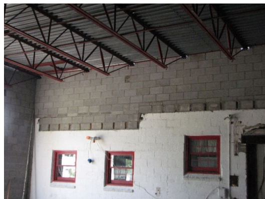
5. Roof joists and deck are hoisted into place
