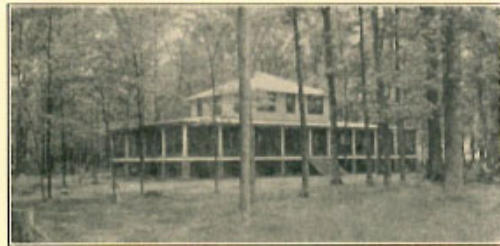
View of Our Club House
