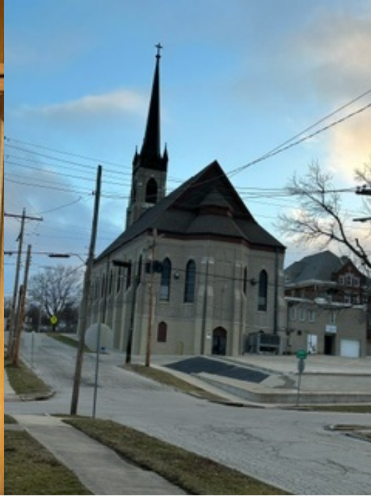
From south looking north across Mason Street.
