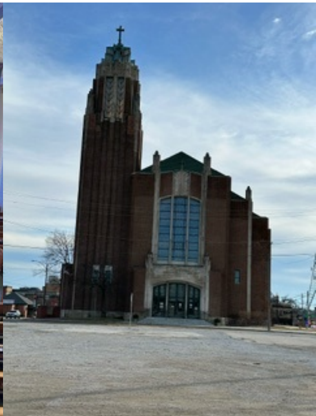
The front of the church which faces north. Photo taken facing south from the parish parking lot located across Chestnut Street.
