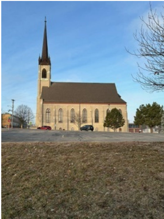
From east looking west near 2 nd parking lot across Mason Street.
