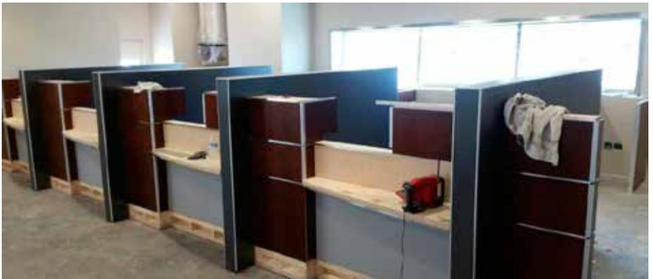
*A lippage control system keeps both pieces of TPT per wall side flush. Walls were installed, and counters assembled.*
