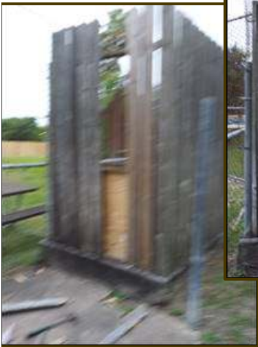
Pool Break in #1 & Repair
