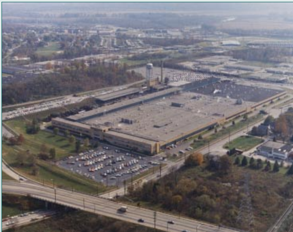
Fairfax Plant: bird's eye view
