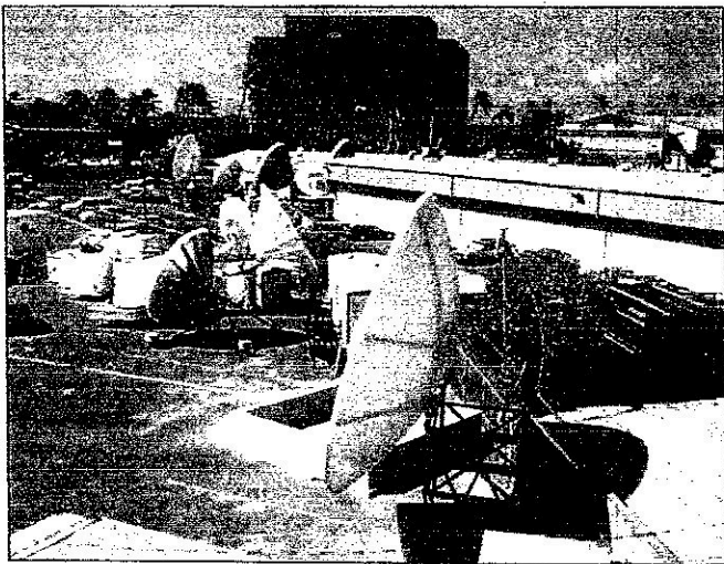
7-meter antenna at Hawaii Overseas Teleport.
