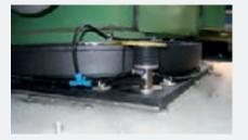
Very robust galvanised proportional valve. Level accuracy is approximately ± 1/10 mm. Suitable for Bilz FAEBI®, FAEBI®-HD and BiAir® air spring insulators.
