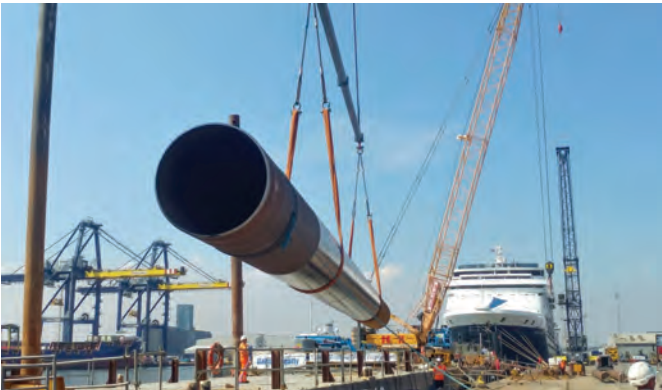
Project Management: Navigator Terminal, Thurrock, Essex
