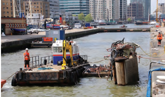
Marine Engineering: West India Dock, London, E14
