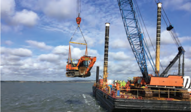
Marine Construction: Lower Hope Nature Reserve, Kent
