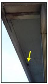
Gable overhang on north end has minor moisture damage
