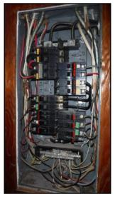
Stab Lok breakers are obsolete
