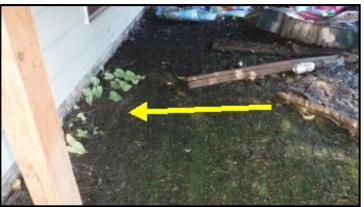
Concrete in perimeter grade slopes toward foundation wall
