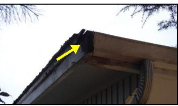
Beam is missing flashing
