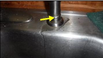
Spray wand leaks at hose connection
