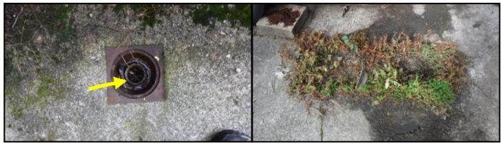
French drain is clogged with debris
