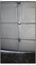
South garage door heavily damaged
