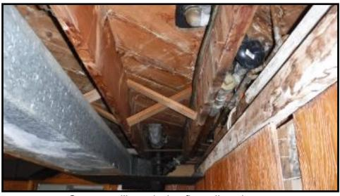
Garage ceiling missing firewall enclosure
