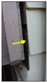
Siding has been cut away and left unflashed for deck attachment
