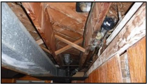
Garage firewall is missing, smoke & fire hazard exists
