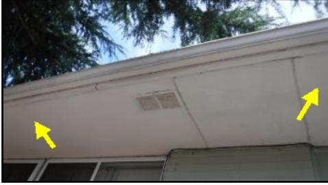
Roof is in need of additional soffit vents
