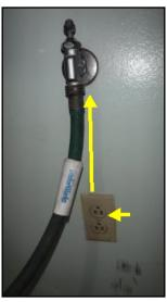
Laundry electrical outlet improperly located and not GFCI equipped
