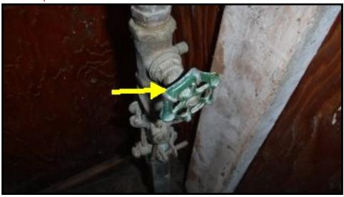
Main shutoff valve is in need of replacement or repair for leaks
