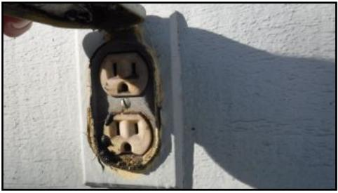
Exterior outlets in are not GFCI protected
