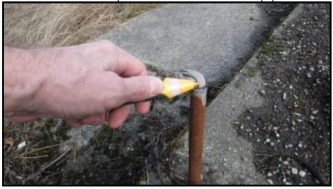
Exposed energized electrical line is a hazard
