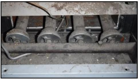
Heat exchanger is in poor condition
