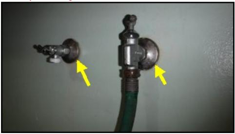
Laundry plumbing valves may be leaking inside wall
