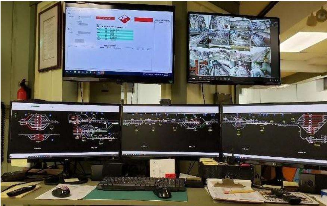
Upper Left / Train Tracker; Upper Right / 16 Video Views of PSRY; Bottom Screens / Display of entire PSRY activity
