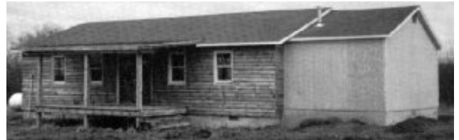
A longhouse built on the reservation
