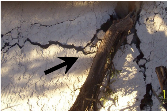
Tree branch embedded into exterior wall from impact
