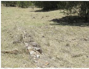
The foundation of an adobe building bulldozed at Mowry, Arizona. Note that the stones are flat. Rough stones would have cracked adobe bricks.
